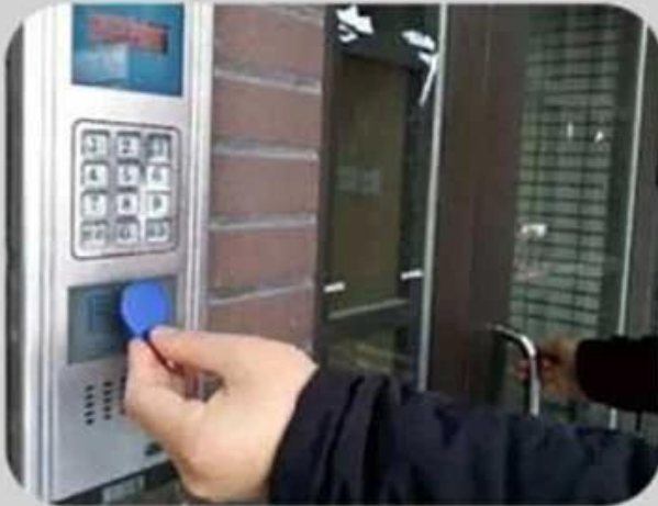
Door Access Control
