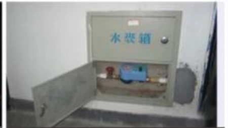
WATER METER BOX
